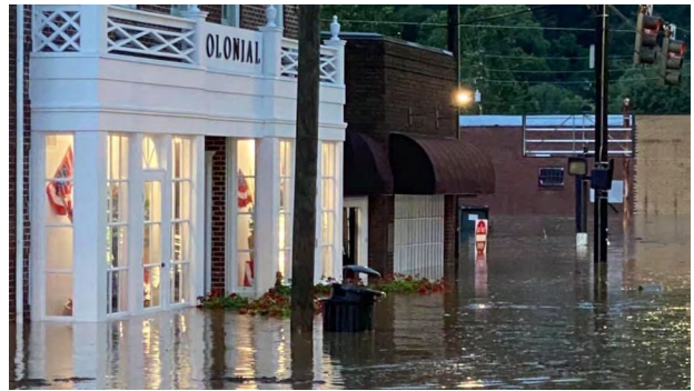
The Colonial Theatre in downtown Canton, N.C., in the aftermath of Tropical Storm Fred, 2021. Courtesy of GoFundMe Fundraiser by Taylor Thompson.
