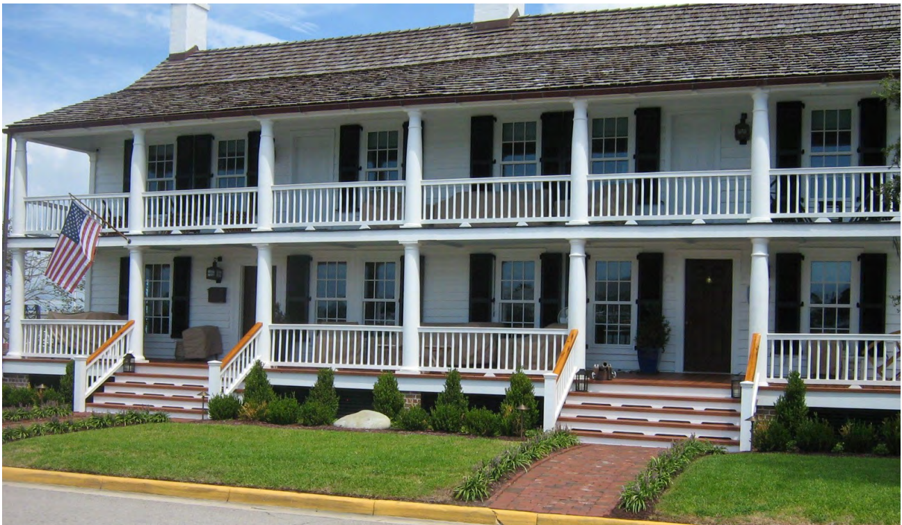
The Town of Beaufort, N.C., and the N.C. Historic Preservation Office worked with the property owners of the Duncan House on Front Street to elevate it above the design flood elevation (base flood elevation plus the required freeboard) in a historically appropriate manner. Top photo courtesy of Filter Design Studio, P.L.L.C.; bottom photo courtesy of Kyle Garner, Town of Beaufort.
